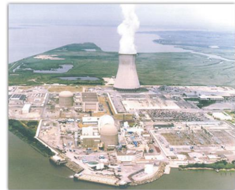
Figure 1: Nuclear Plant With PHoenix™ Skid installed on EHC System
